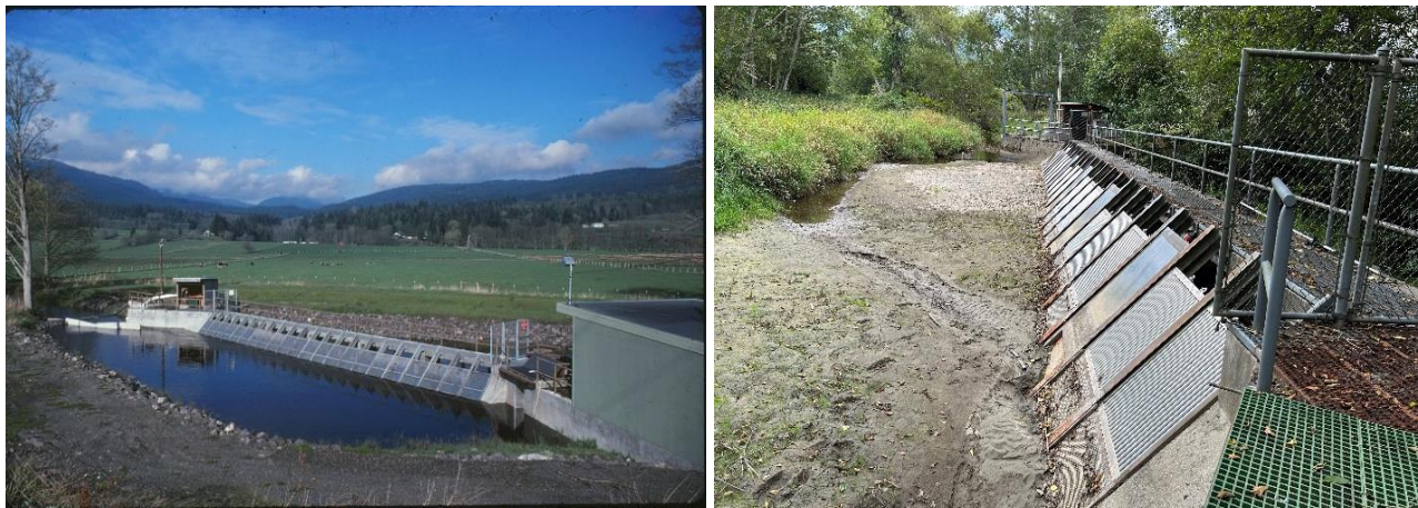
Figure 2. Snow Creek permanent full spanning weir newly constructed (circa 1978, photo left), and sediment accumulation in front of weir September 2023.
