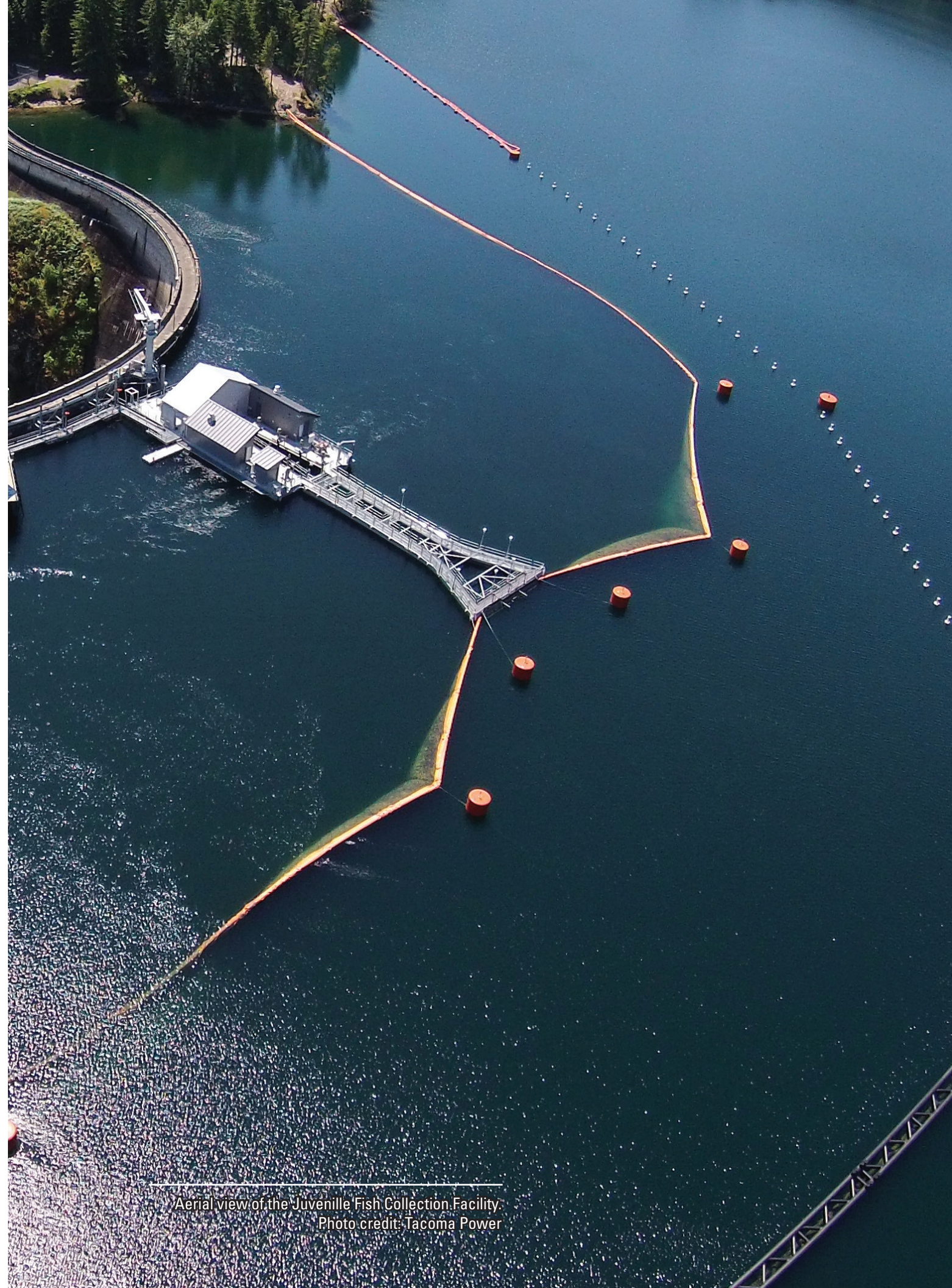
The FSC is connected to Cushman No. 1 Dam, and the NTS is connected to, and funnels fish from the reservoir into, the FSC. Captured fish are removed and released into the North Fork Skokomish River downstream of Cushman No. 2 Dam.
