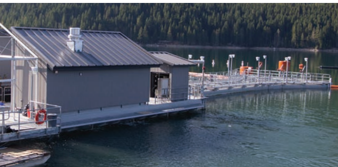
The FSC is connected to Cushman No. 1 Dam, and the NTS is connected to, and funnels fish from the reservoir into, the FSC. Captured fish are removed and released into the North Fork Skokomish River downstream of Cushman No. 2 Dam.
