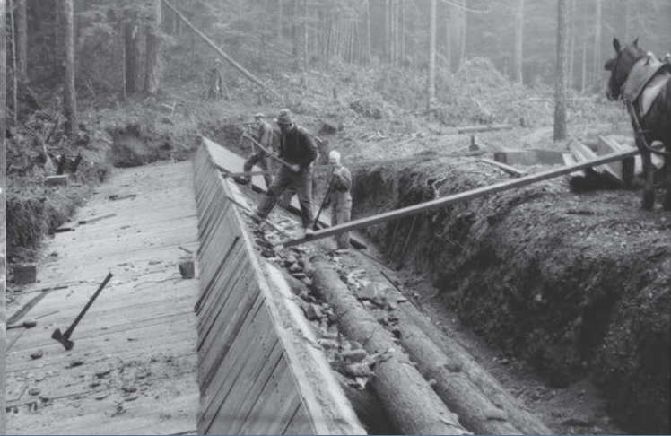
FILLING AND PLANKING LOG CRIB DAM FROM EASTERN EXTENT OF DAM, FACING WEST. December 1926 - Cushman No. 1 Hydroelectric Power Plant, Spillway, North Fork of Skokomish River.
