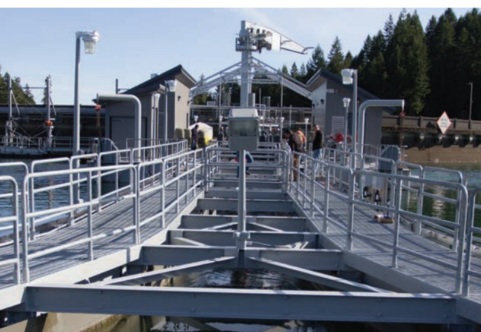
The FSC is connected to Cushman No. 1 Dam, and the NTS is connected to, and funnels fish from the reservoir into, the FSC. Captured fish are removed and released into the North Fork Skokomish River downstream of Cushman No. 2 Dam.
