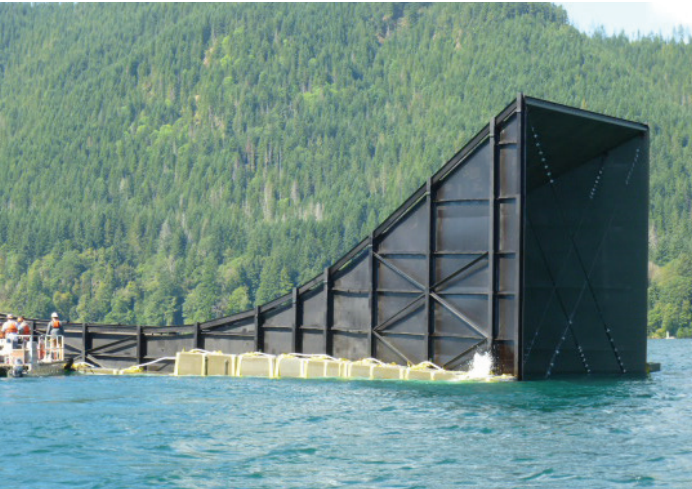
The two structures were joined to make up the juvenile fish collection facility used to capture juvenile salmon as they try to leave Lake Cushman on their way to the ocean.
