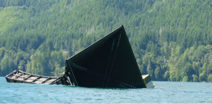
The Net Transition Structure (NTS) flipping over in Lake Cushman in preparation for connecting it to the Floating Surface Collector (FSC).
