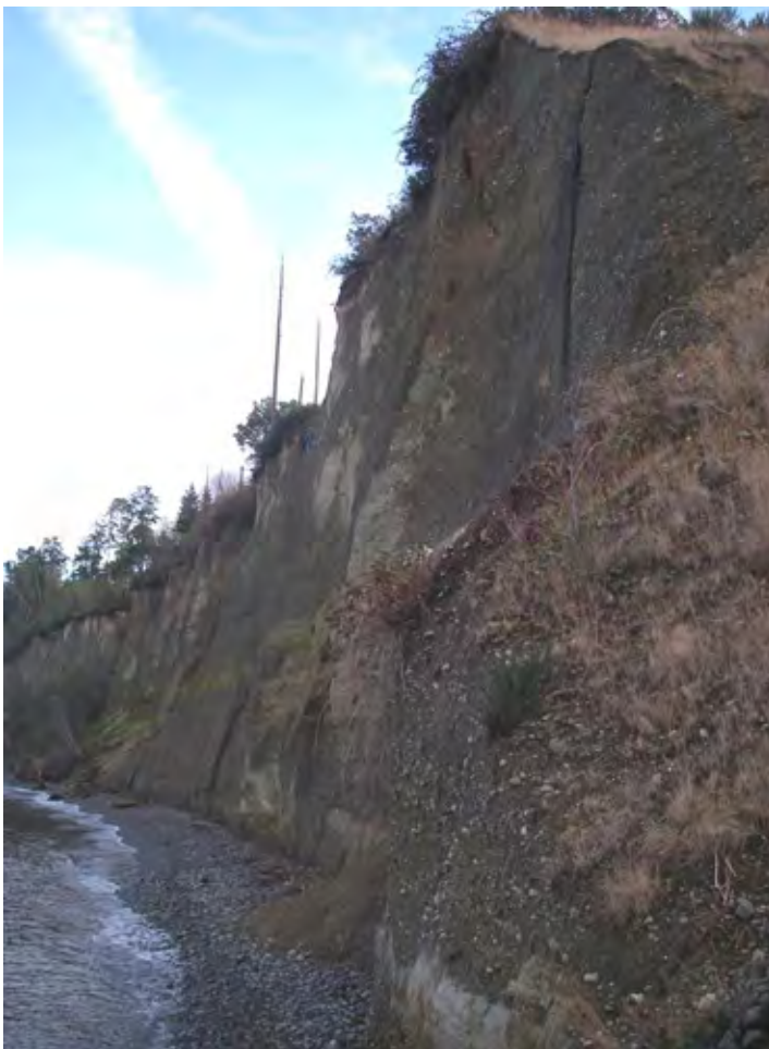
Current site conditions east end cell 304
