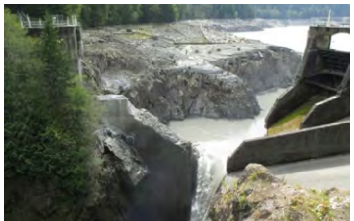
Glines Canyon Dam, 2012
