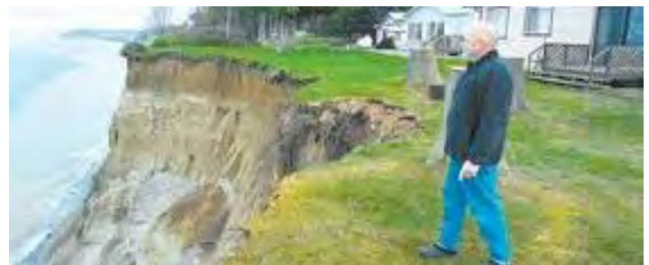
Bluff erosion in Clallam County
