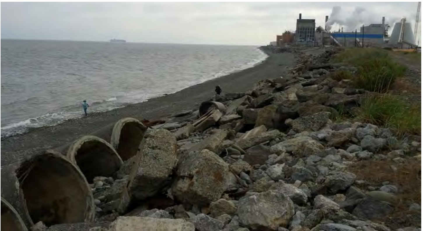
Extensive shoreline modification in Clallam County
