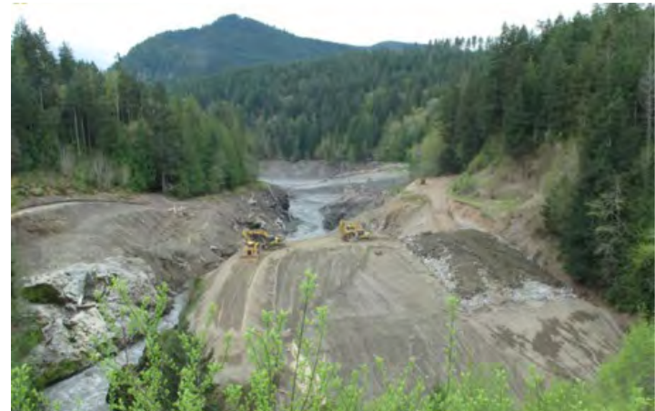
Elwha Dam Removal, 2012
