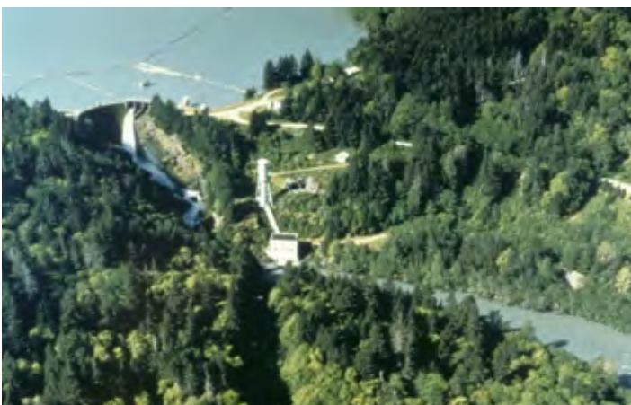
Glines Canyon Dam before removal
