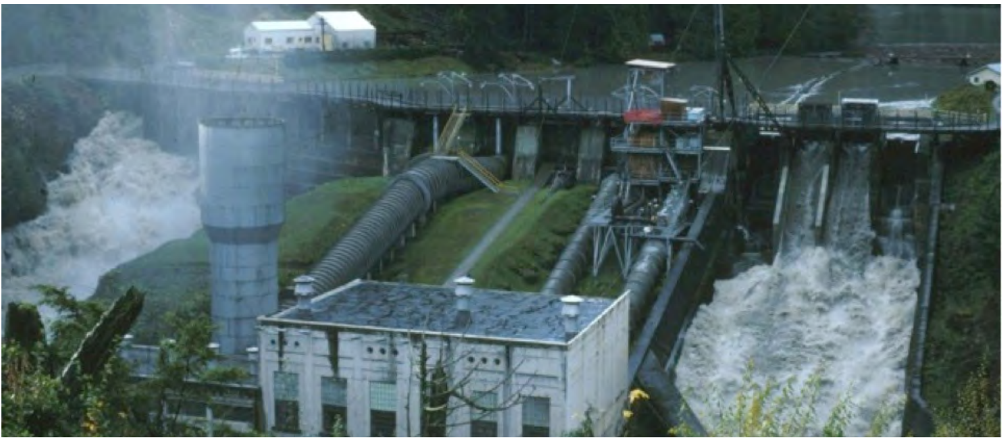
Elwha Dam before removal
