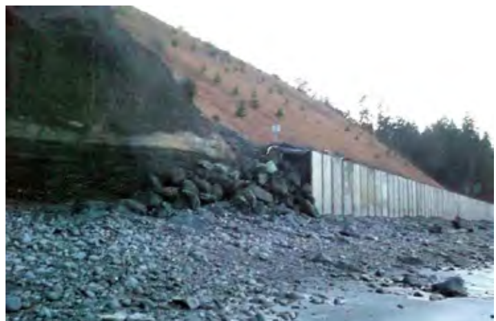
Completed seawall-Port Angeles Landfill
