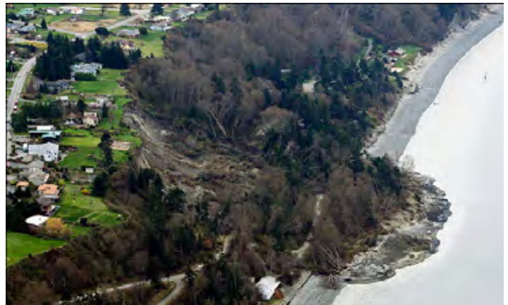
Whidbey Island Landslide, 2012
