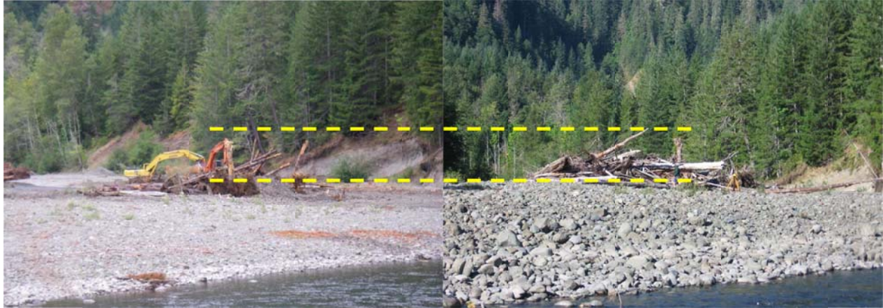
Figure 4-4. Example of changes to a gravel bar where a logjam had been built in Phase 1. On average gravel bar heights increased 2.4 feet through the project reach. Maximum accumulation height on structure #5 (shown) was 6.6 feet. From Geiger (2015).
