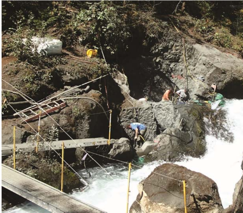
Figure 4-11. Workers completing modifications to Little Falls to improve passage for upstream migrants.
