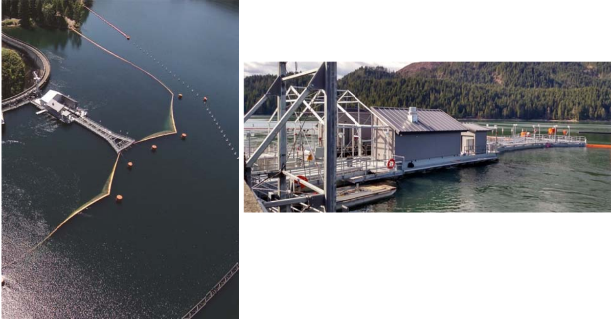
Figure 4-10. Left – Aerial photo showing the Floating Surface Collector (FSC) in place at the lower end of the upper reservoir and attached to the upstream face of the dam. The guide nets, arranged roughly in a “W” shape to help guide downstream emigrants to the upstream opening of the FSC, are also seen. Right – The FSC structure as seen from the rim of the dam.
