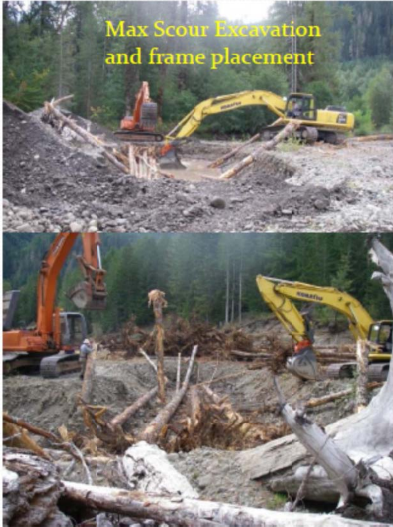
Figure 4-3. Construction of logjams in Phase 1 in the Holman Flats reach.
