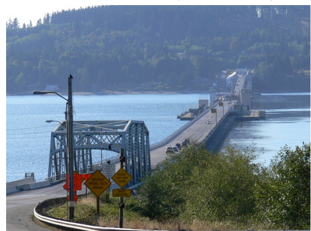
Hood Canal Bridge. Photo by Flickr user Ann & Peter Macdonald
