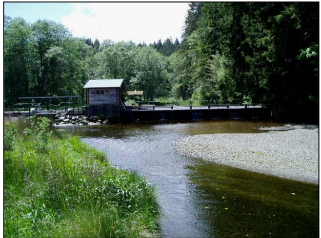
The University of Washington facility, with monitoring station BB01 in the foreground
