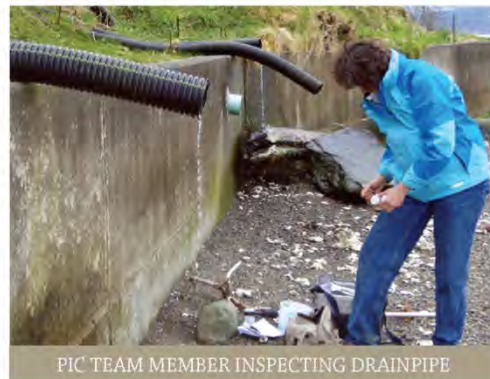
PIC TEAM MEMBER INSPECTING DRAINPIPE
