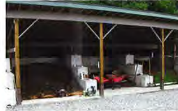
Manure composting facility. Photo from Mason Conservation District.
