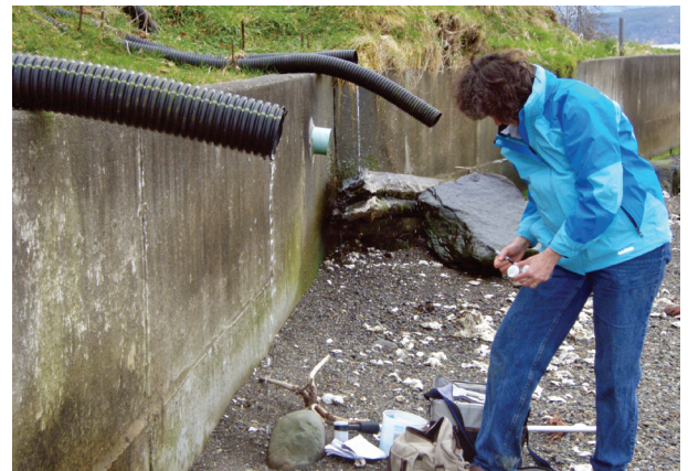
PIC TEAM MEMBER INSPECTING DRAINPIPE
